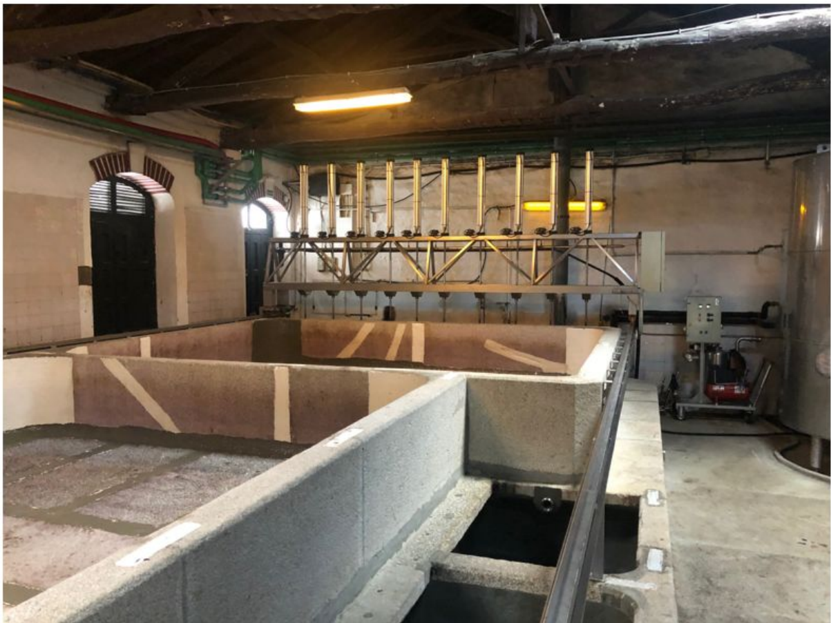
Robotic lagares. Here, the lagares are made from granite.
